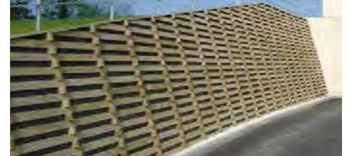
Cribblock retaining wall
