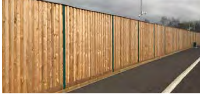
Typical Acoustic Fence
